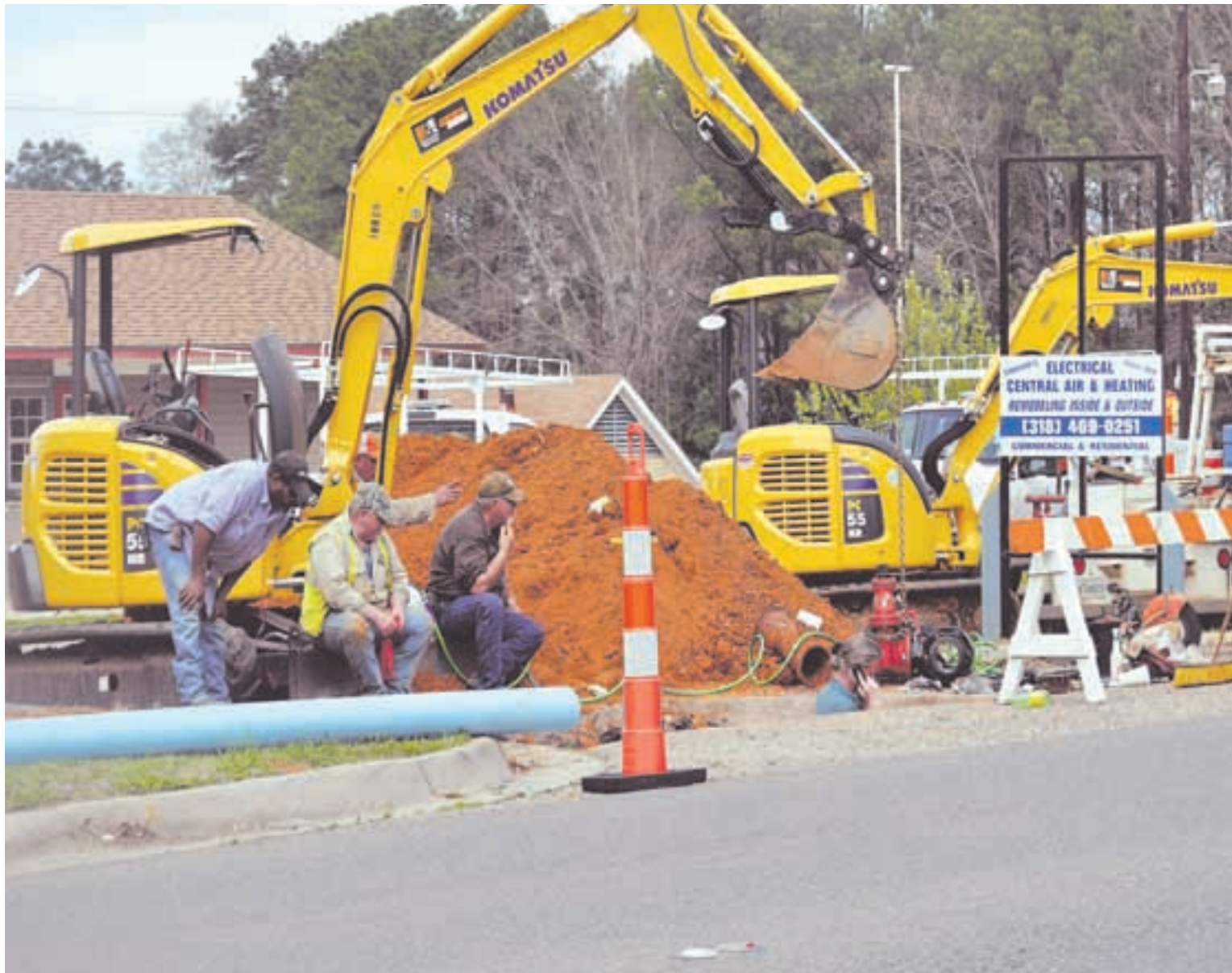
Eric Lee, City of Minden Distribution and Collection supervisor, checks on progress at the bottom of a hole at the intersection of Myers and Lee streets where contractors are replacing a water valve. Bonnie Culverhouse/Press-Herald
