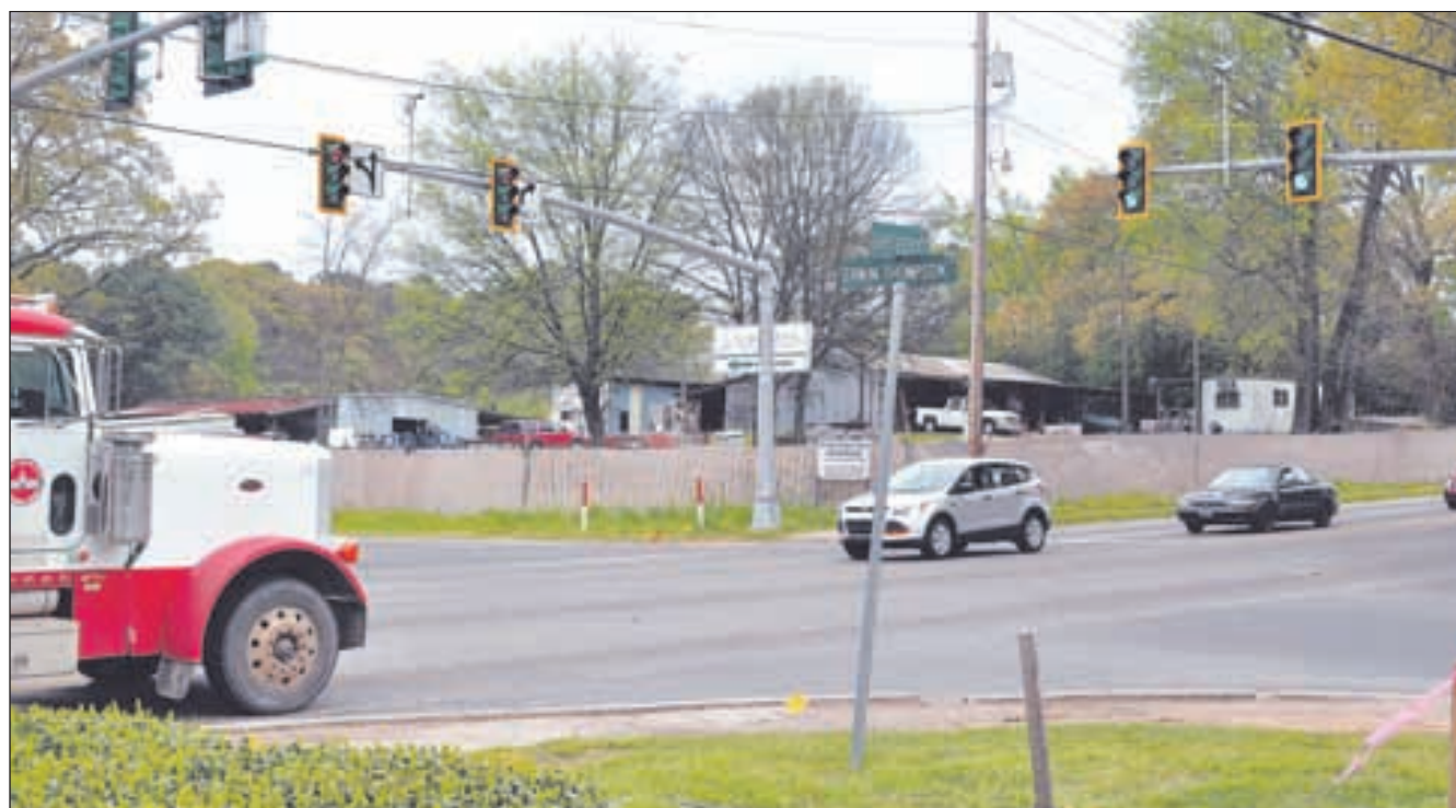
DOTD has been issued a "notice to proceed" for improvements at the corner of U.S. Hwy. 80 (Shreveport Road) and Erwin Thompson Drive. District 04 Director David North says that will include expanding the radius on the turns for 18-wheelers going to Fibrebond Corporation. North says the work is very involved. "They will have to take out the curb and add a segment of pavement, wrap around and recurb it," he said. Bonnie Culverhouse/Press-Herald
