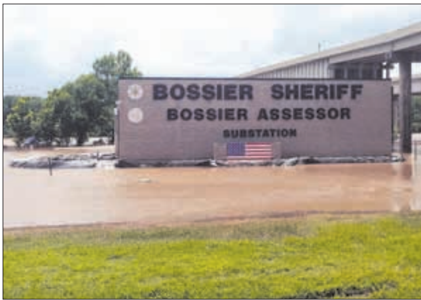
Water levels on the Red River has started to fall. The American flag on the side of the substation is now showing. Only a few strips at the top was visible when the river was at its highest. Courtesy Photo/Bossier Parish Sheriff's Office
