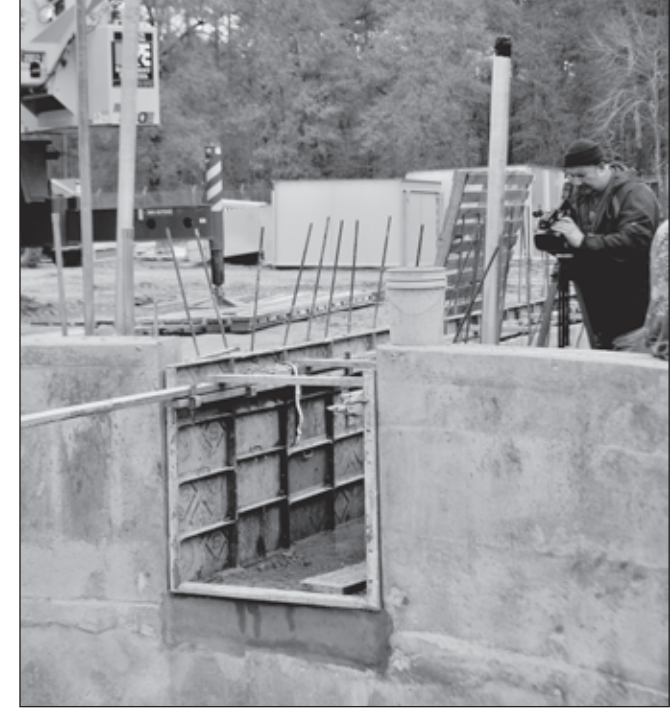
The track shown above will move the prepared M6 propellant into the contained burn unit for destruction. ESI officials say the burn will only take seconds, but as the pollution abatement system scrubs the gasses emitted from the burn, the entire process will take about 15 to 20 minutes, with the goal of conducting three burns of about 880 pounds per hour. Michelle Bates/Press-Herald
