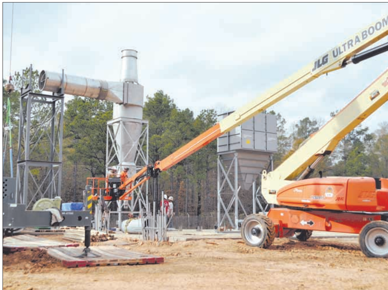
Crews work to erect the pollution abatement system at Camp Minden, Area I. The abatement system will scrub the gasses coming from the contained burn unit that will destroy nearly 16 million pounds of M6 artillery propellant and some 800,000 of clean burning ignitor. Michelle Bates/Press-Herald
