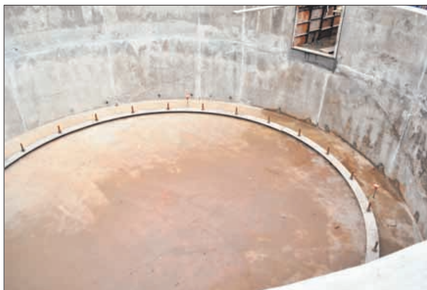
The contained burn unit on its way to Camp Minden from Oklahoma is 24 feet in diameter, 110 feet tall and weighs 200 tons. The base of the unit shows the sheer size of the unit. Michelle Bates/Press-Herald
